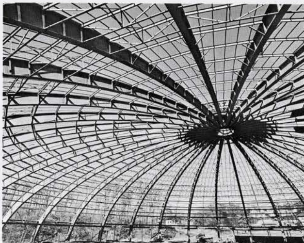
This is the structural steel framework for a college sports arena. Because of the strength possible with steel design, there are no columns to obstruct spectators' vision.
