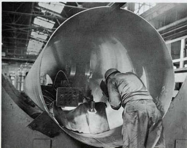
Large-diameter steel pipe is made by welding curved plates.
