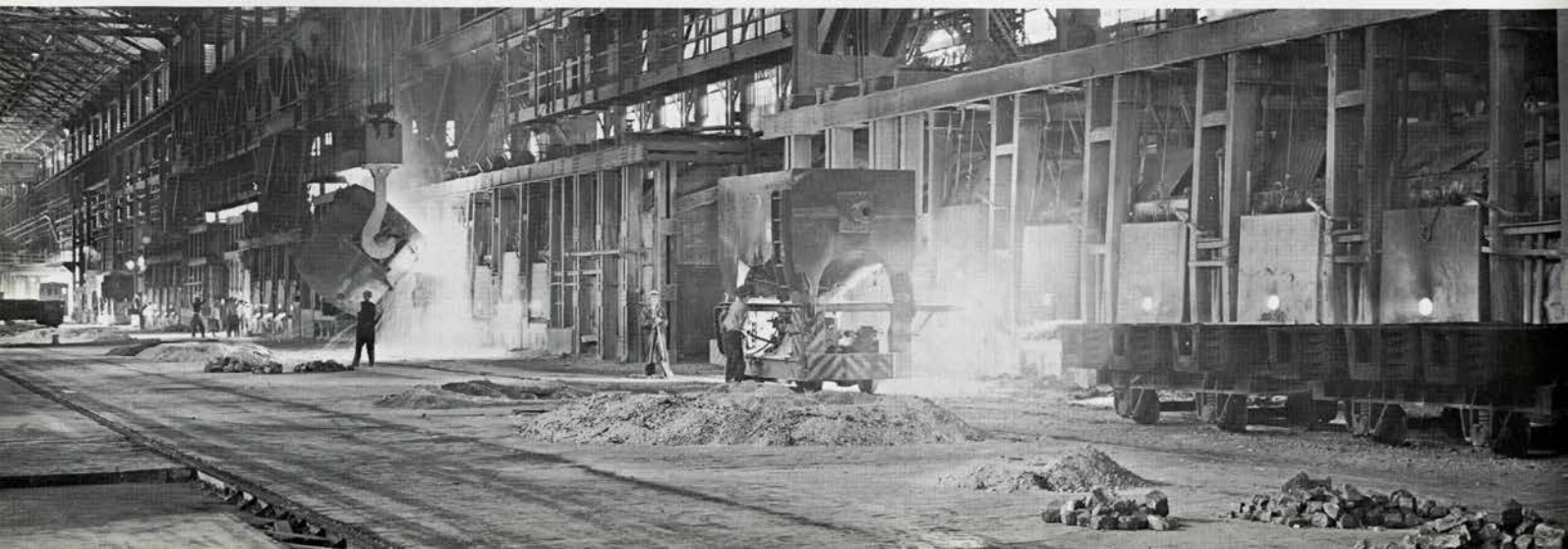
Open-hearth charging floor at the Saucon Division of the Bethlehem Plant, where steel is made for rolling into structural shapes.
